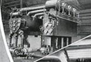
Quietness and absence of vibration and moving parts characteristic steam-jet units. Water, the refrigerant, is evaporated at a high vacuum and the vapor is compressed by steam-jet nozzles. The water chilled by this evaporation is the cooling medium. The condenser may be of surface or barometric type. Exhaustor & B isolates simply connect. Sizes from 10 tons upward.
